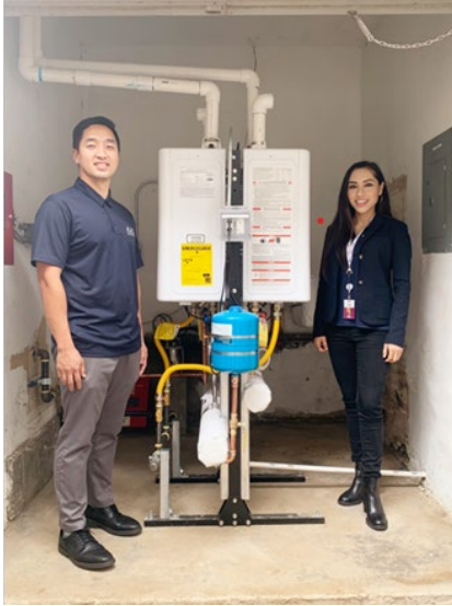
Figure 38. SoCalREN Multifamily Program AMP Visit
