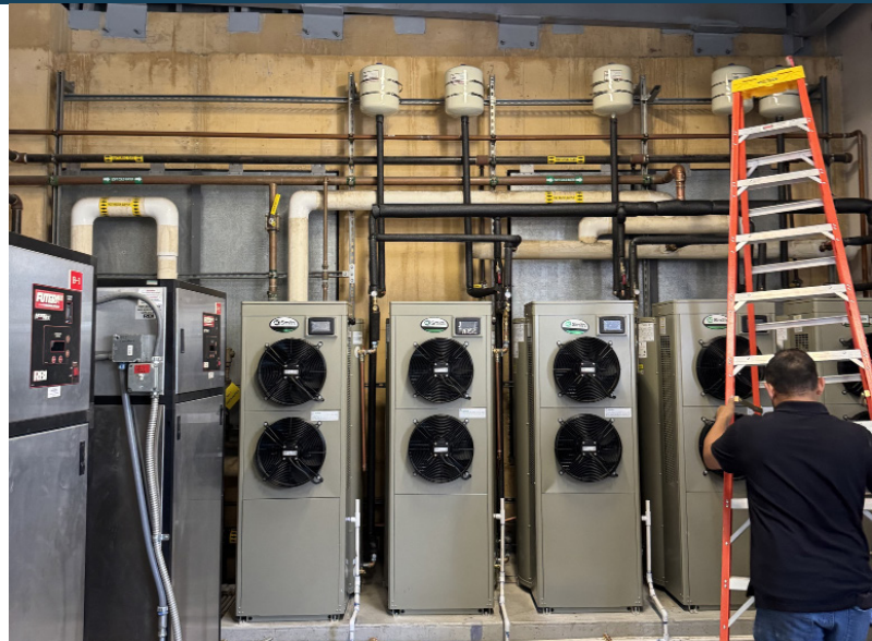
Picture: Heat pump water heaters installed in UCI Health medical facilities, Orange, CA.
