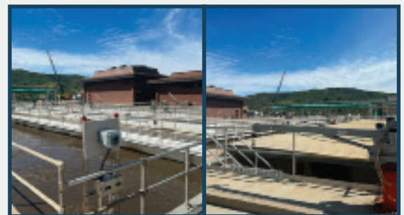
Pictured: The aeration basins at the City of Simi Valley's Water Quality Control Plant post-installation
