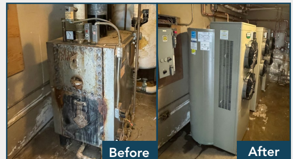
Before and after photos of one of the water heater replacements
