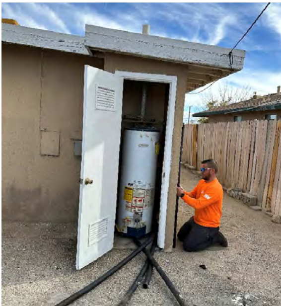
Figure 3. Multifamily Program Contractor at Project Site
