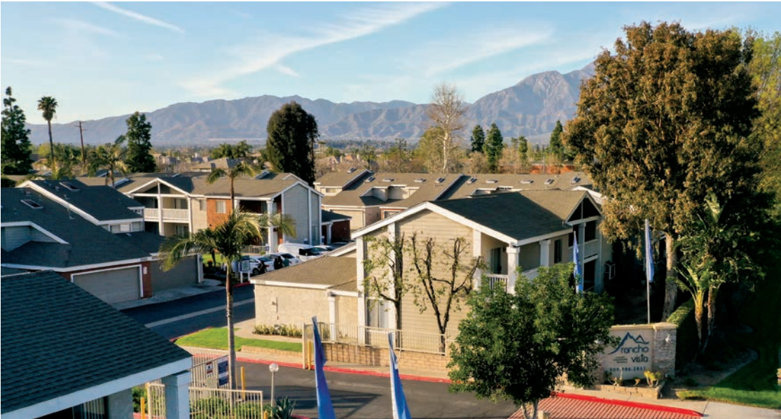
Rancho Vista Apartments in Ontario (San Bernardino County) participated in the SoCalREN Multifamily Program, completing an upgrade to exterior lighting, delivering energy savings and greater security for residents.
