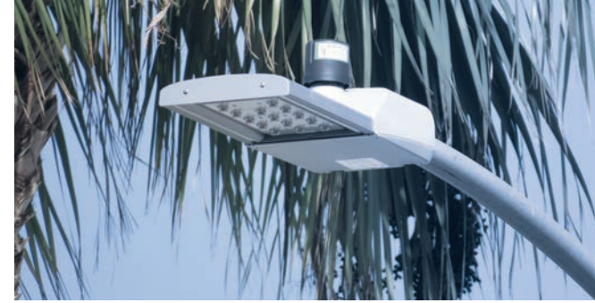
LED street light upgrade in The City of Orange
