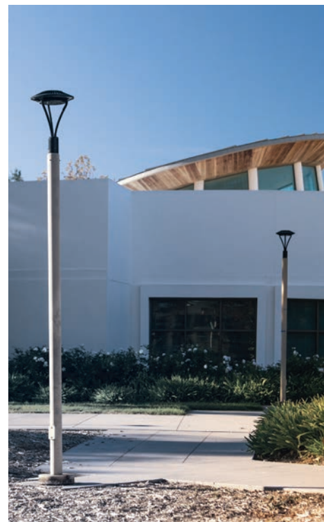
Interior and exterior lighting was improved at the Simi Valley Senior Center.
